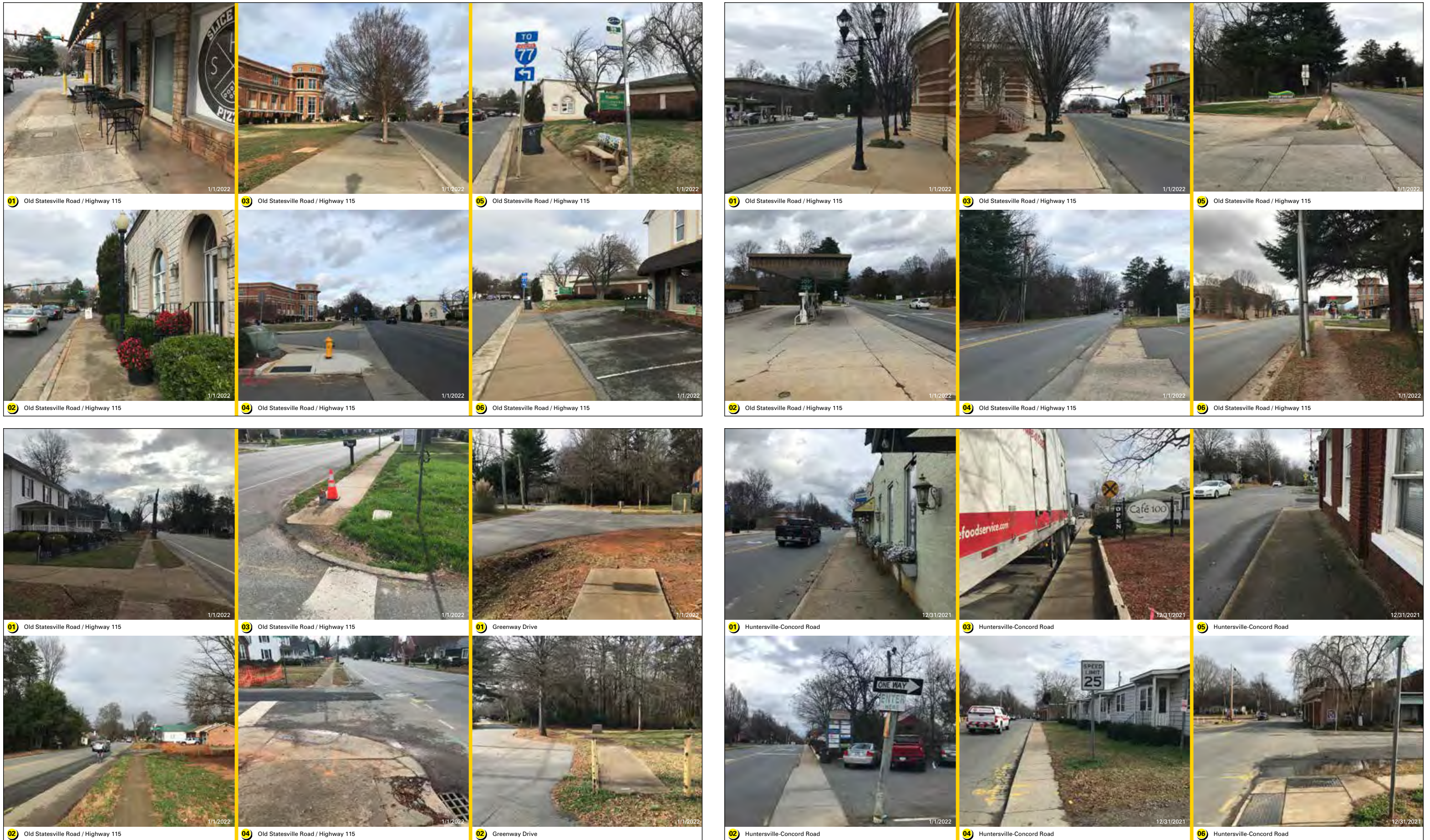
FIGURE 31: Preliminary Assessment - Infrastructure: Downtown Sidewalks and Streetscape (Existing Conditions).
