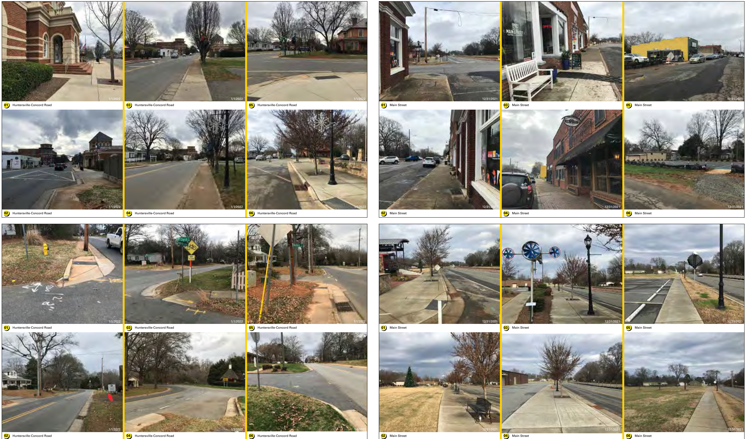
FIGURE 32: Preliminary Assessment - Infrastructure: Downtown Sidewalks and Streetscape (Existing Conditions).
