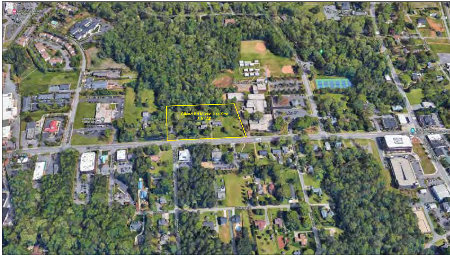
FIGURE 20: Gillead Road Mixed-Use Project - Huntersville, NC: Project Site Location and Context.
